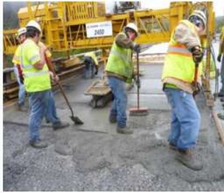
Ozyildirim, Celik and Nair, Hari Krishnan.(2010). (b) Placing overlay [Digital Image] Charlottesville, VA: Virginia Transportation Research Council
