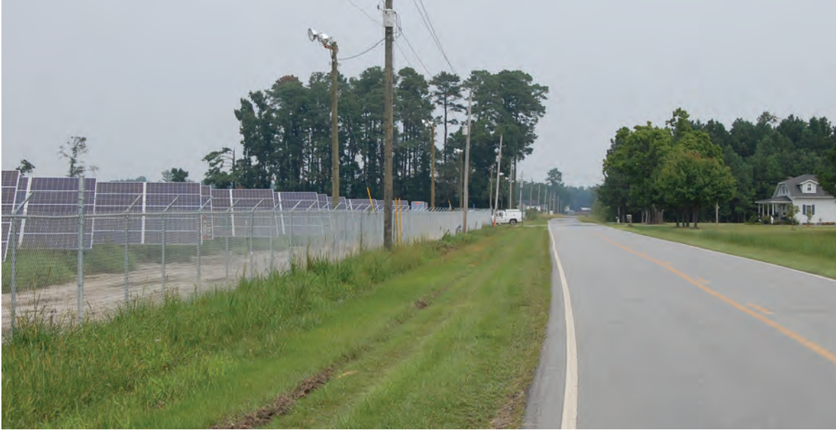
Solar farms, such as this one in Beaufort County, can have significant visual impacts, particularly without any setback or buffering requirements.
