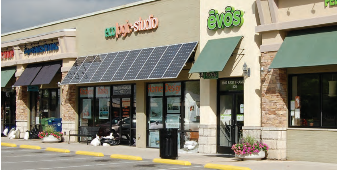
Building-integrated solar panels—in this case, a PV awning.
