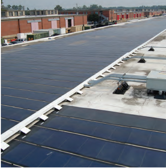
Commercial-scale solar commonly makes use of the large, flat roofs of today's commercial buildings. PV or thermal panels may be installed flat or pitched to increase energy production.
