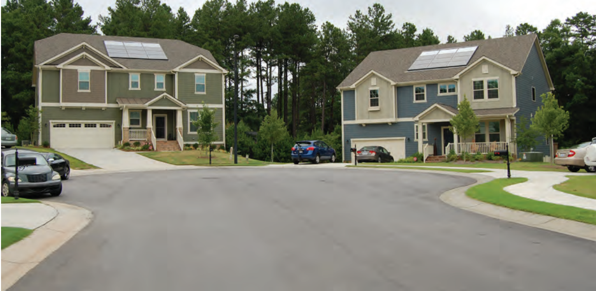
Residential-scale solar provides some or all of the energy needs of a residence. These residential solar installations in Durham incorporate PV and thermal.
