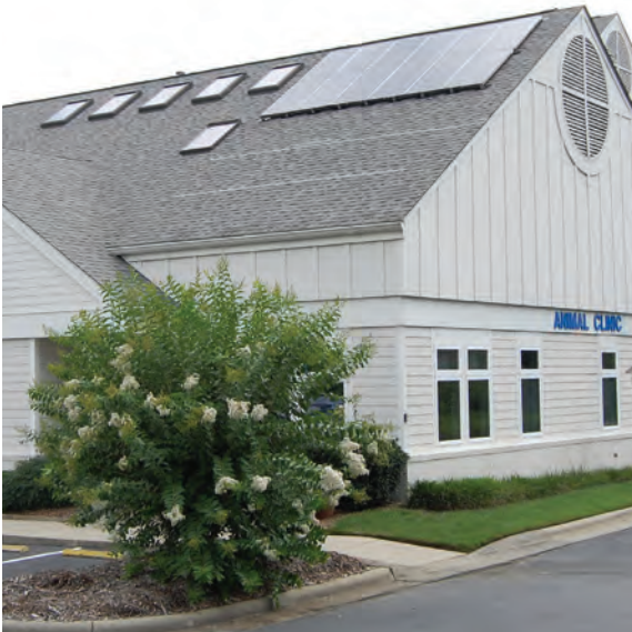
Flush-mounted solar panels on a pitched roof.
