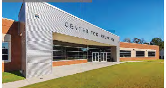
EDGECOMBE COMMUNITY COLLEGE CENTER FOR INNOVATION
