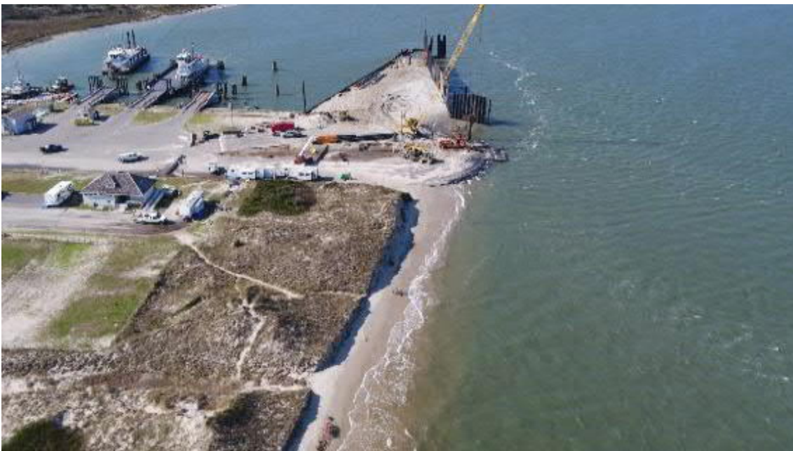
Photos of South Dock Erosion
